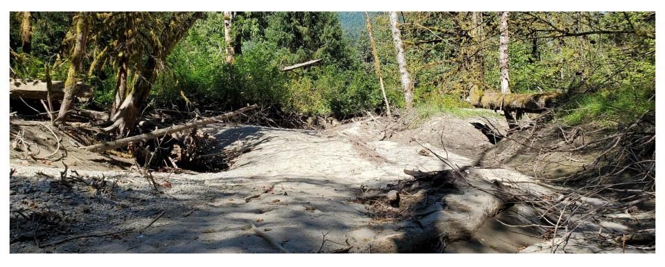
Brandt Channel – Tributary to Indian River 1980 Constructed Groundwater Chum spawning channel Changes in Indian River Flows deposited approx. 2 meters of sand/gravel
