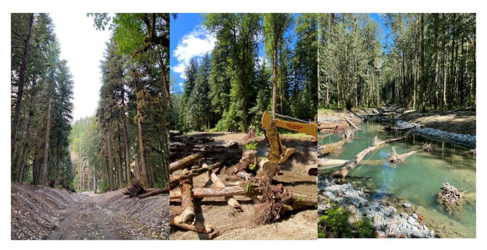
Summer 2022 - Constructed sockeye and coho spawning channel Fall 2022 observed sockeye chum moving back into channel
